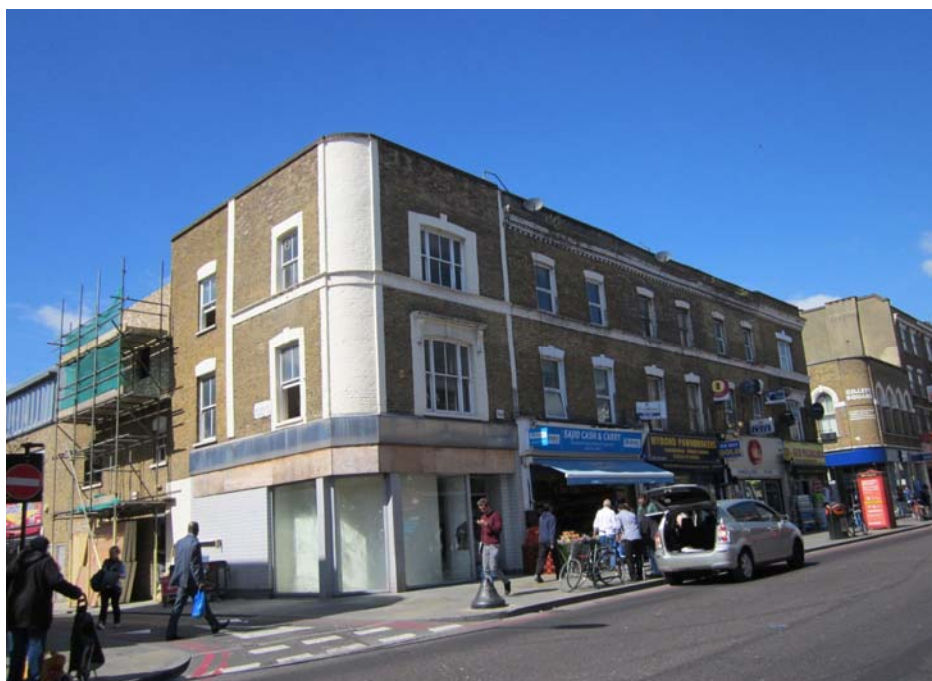
Figure 36: Nos 71-81 Kingsland High Street
