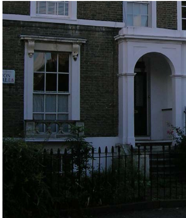
Figure 35: Replacement balconies in concrete in Albion Square
