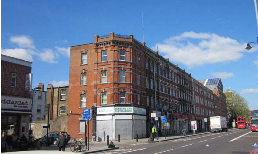
Figure 43: The tall terrace at Nos.19-47 Stoke Newington Road
