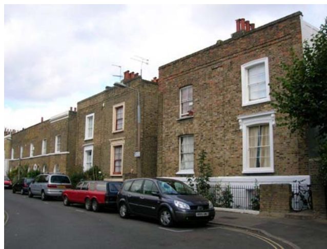
Figures 20, 21 & 22: Cottages in Albion Terrace
