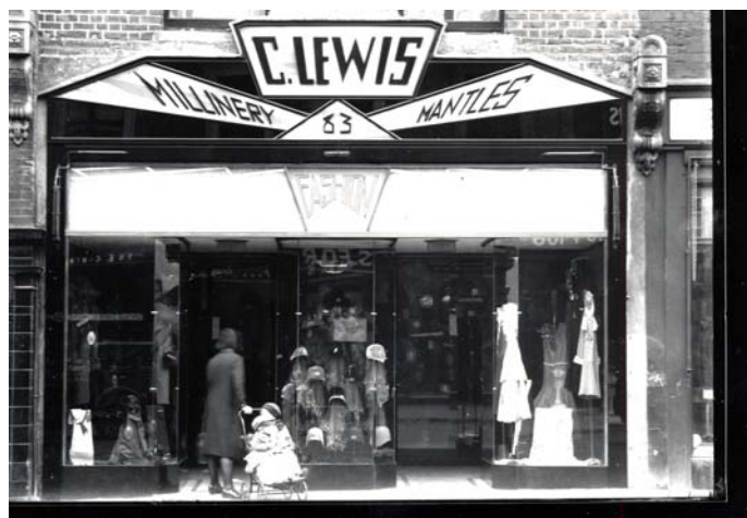
Figure 37: Caplan Lewis, Milliners at No. 83 Kingsland High Street c. 1934 an Art Deco shop front now demolished
