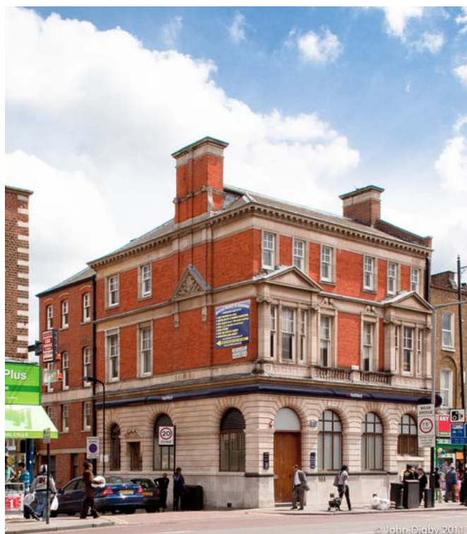
Figure 17: No. 74-76 Kingsland High Street, a locally listed building
