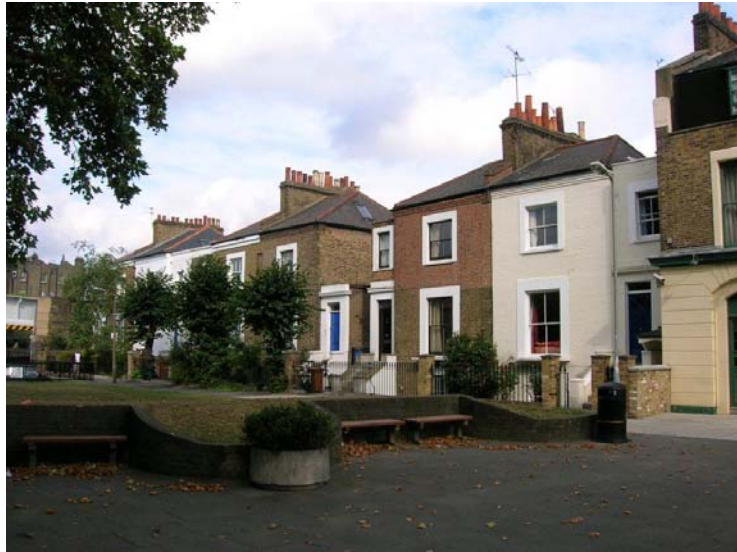
Figure 23: Nos. 262-266, Haggerston Road
