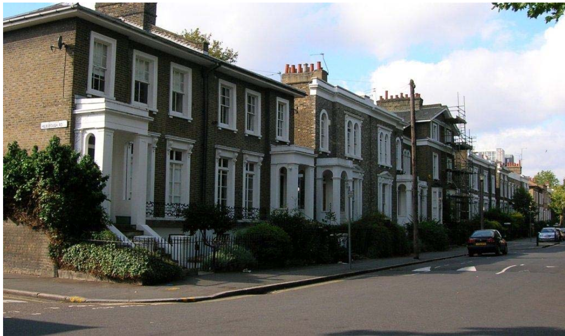
Figure 8: View of houses on the south side of Albion Square
