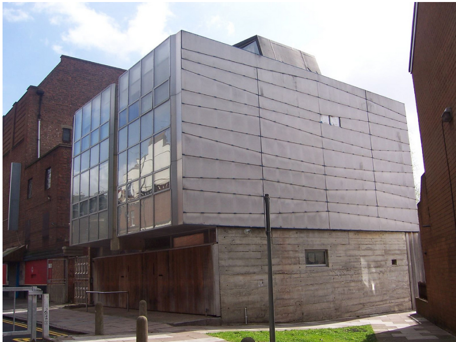
Figure 56: No. 1 Truman's Road, a locally listed building
