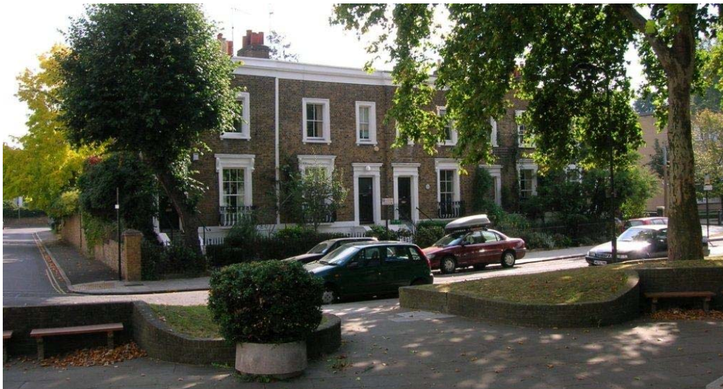
Figure 24: Nos. 250-258 Haggerston Road
