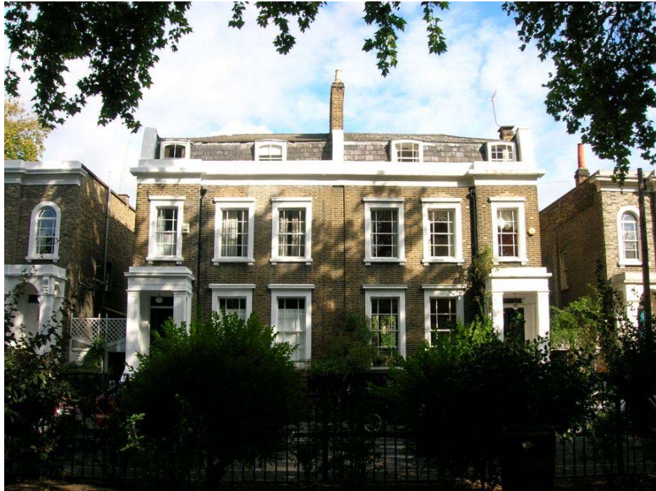
Figure9: Nos. 17 & 18 Albion Square with mansard roof on north side of the square.
