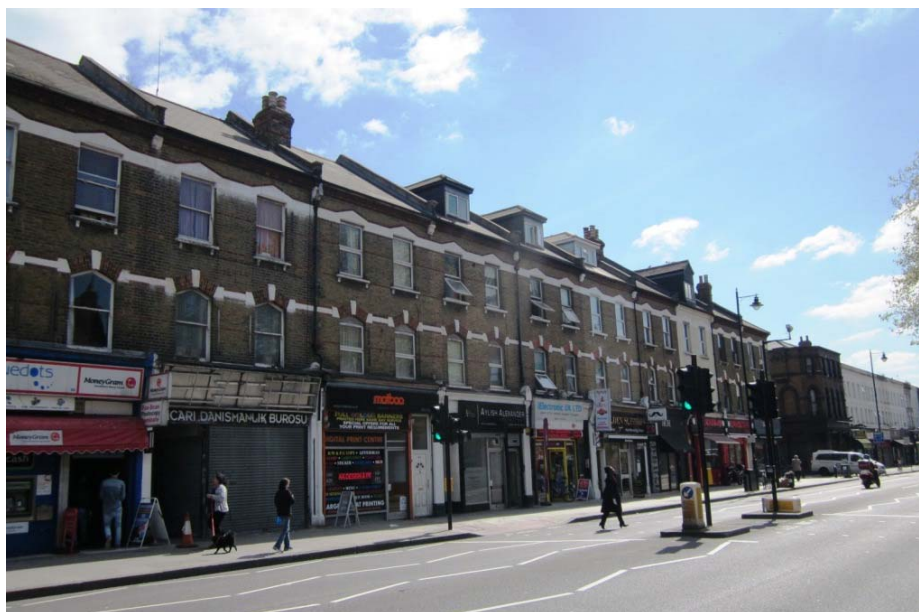
Figure 2: Nos. 68-50 Stoke Newington Road a well preserved terrace
