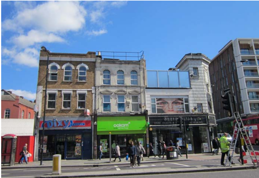
Figure 15: Nos. 2-8 Kingsland High Street
