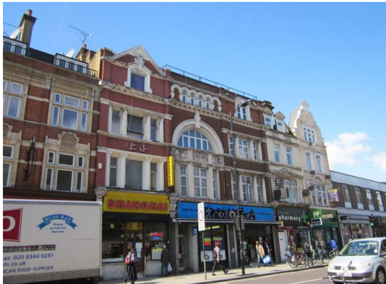
Figure 35: Nos. 39-49 Kingsland High Road
